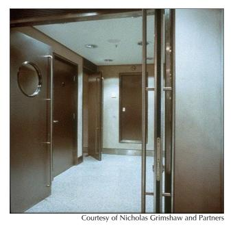
**Figure 15** Stainless steel wall trims and skirting
