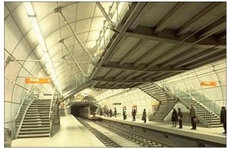
*Figure 6* Stainless steel hangers and struts support the mezzanine
