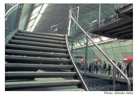
Handrails to the staircase and mezzanine areas are fabricated from 50 mm stainless steel tubes, polished to a mirror finish. These are fixed to balusters at 1.2 m centres by a welded 10 mm plate projecting from a post cap (Figure 12). A threaded spigot joins the post cap to the
