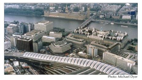
**General** The new International Terminal at Waterloo (Figure 1) is located to the west of the existing Waterloo mainline station and replaces the old Victorian brick vaultings. It comprises a four-storey concrete viaduct accommodating an underground car park, the arrivals, departures, offices and at the top level, just under the roof structure, the train tracks (Figure 2).
